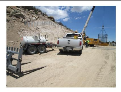
**Photo 2:** During rebar cage installation at Steel Pole 42, water was utilized for dust suppression (MM AQ-1) and fire safety tools (Pulaski, shovel, etc.) were observed staged on site in accordance with MM FF-1.
