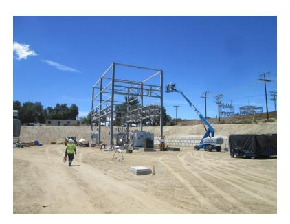
**Photo 5**: Crews were observed working on the 69kV Circuit Breaker Frame at the Boulevard Substation Rebuild. Visual screening was observed in good working order in accordance with MM VIS-3a.
