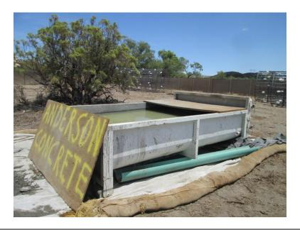
**Photo 1:** Concrete washout basins were observed in good working order in accordance with the project SWPPP and MM HYD-1.
