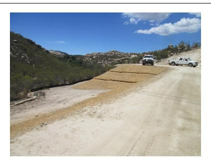
**Photo 3:** SWPPP BMPs (MM HYD-1), including straw wattles and silt fencing were observed in good working condition at Steel Pole 42.
